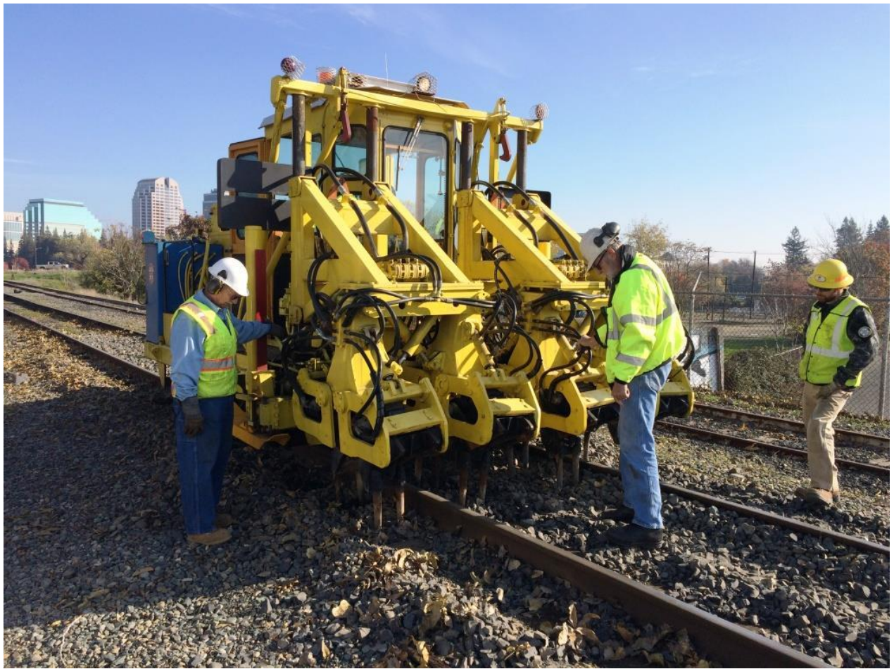
Alan directs Mike F. in the tamper as Clem and Chris M. manually operate the actuators for the work-heads
