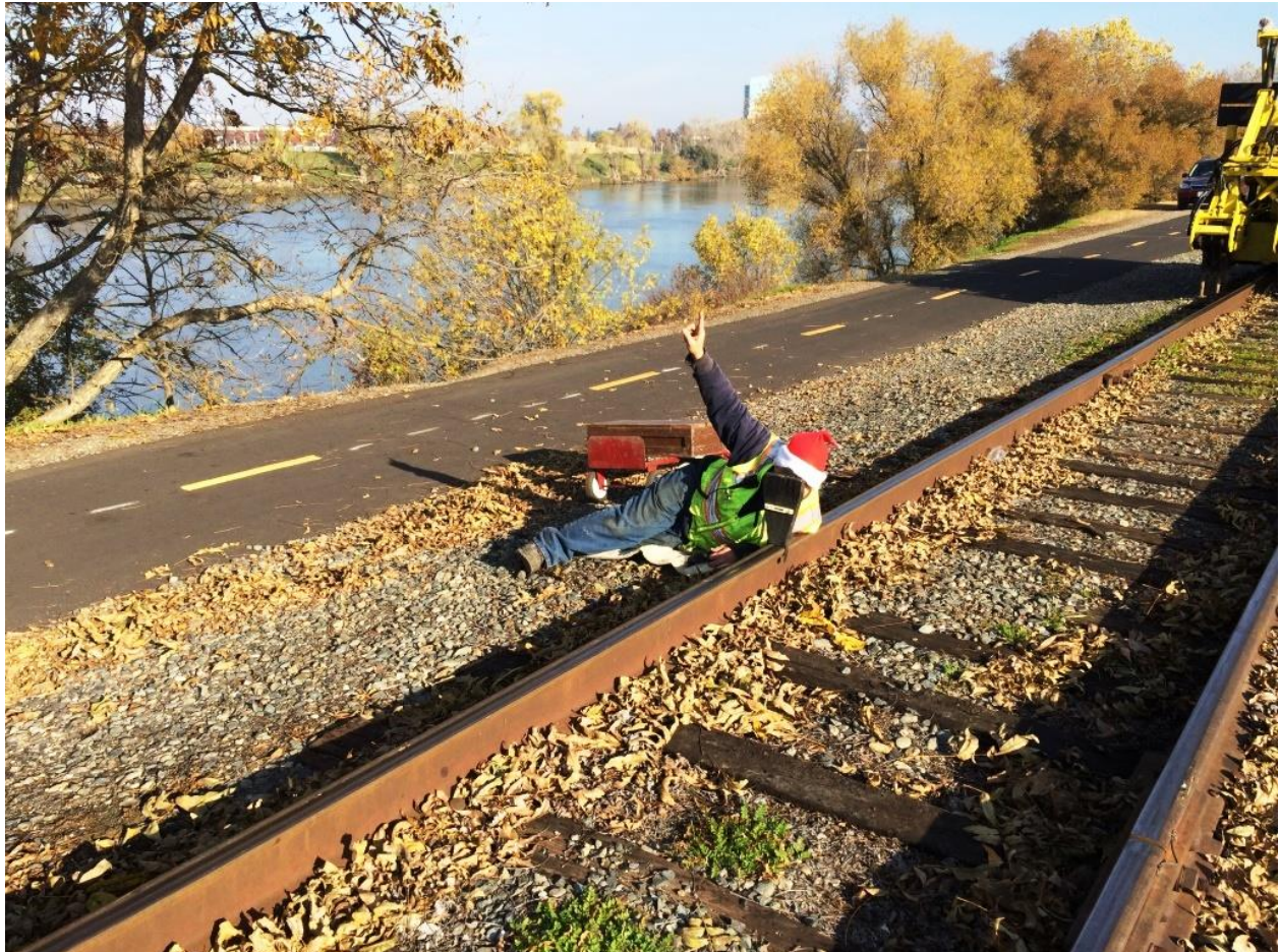
Joe peers through the "rabbit" towards the "spot-board" to measure the raise and directs the Team manning the jacks
