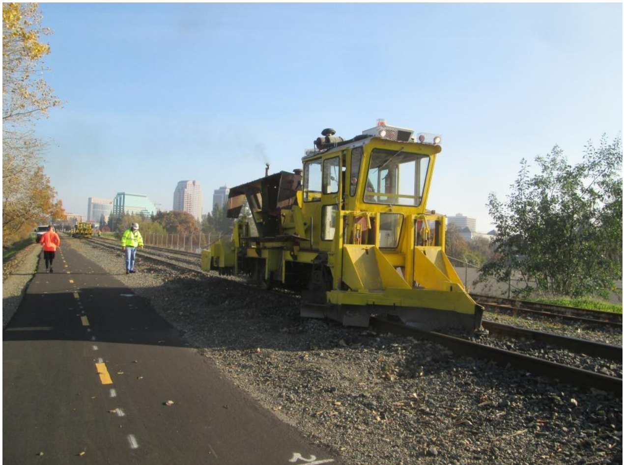
Chris C. in the regulator plows windrows of rock
