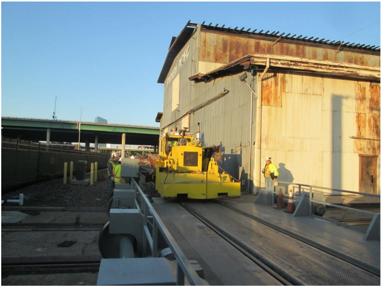
The ballast regulator is deployed
