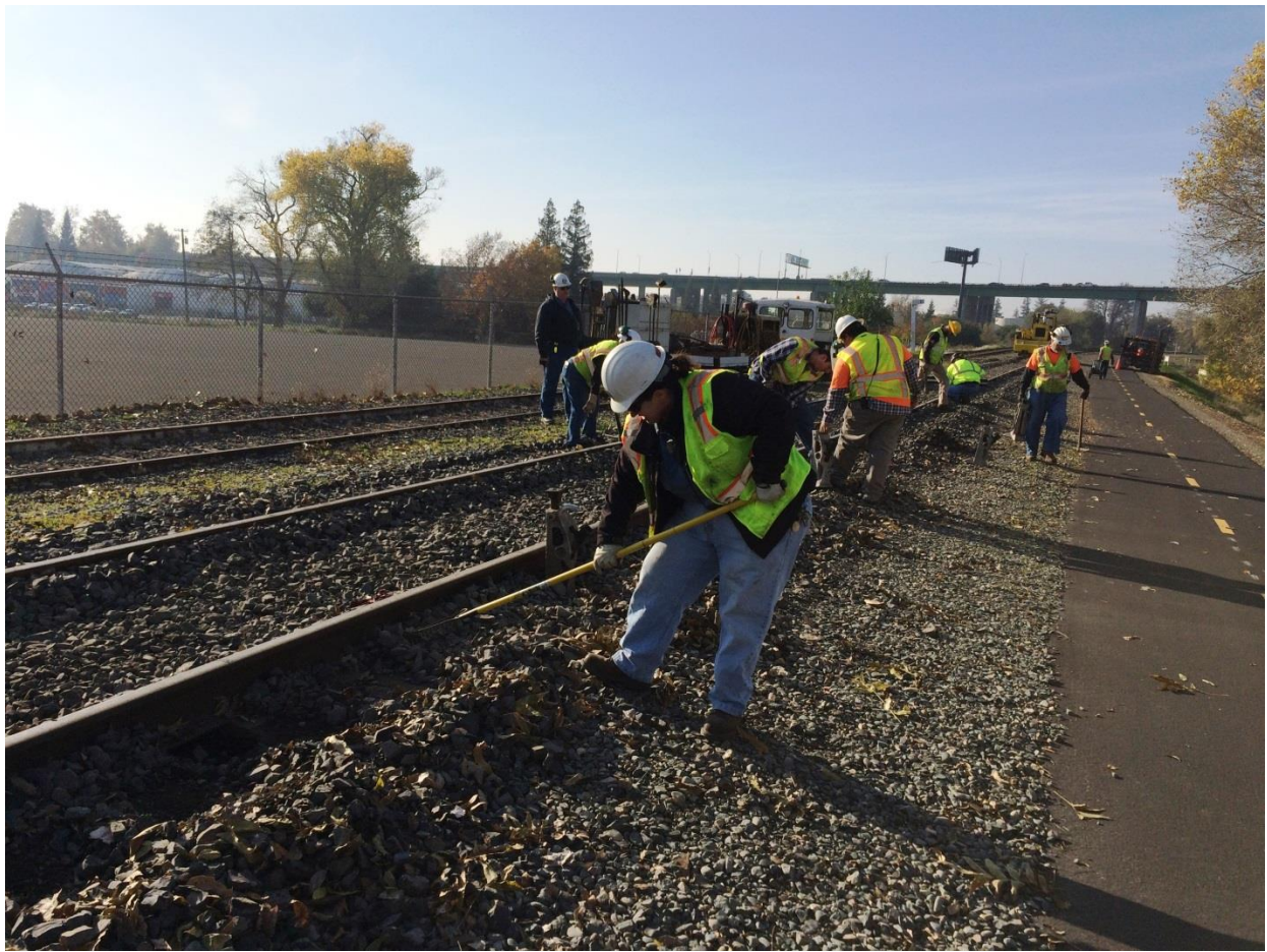
Heather and the Team prepare the rails for raising
