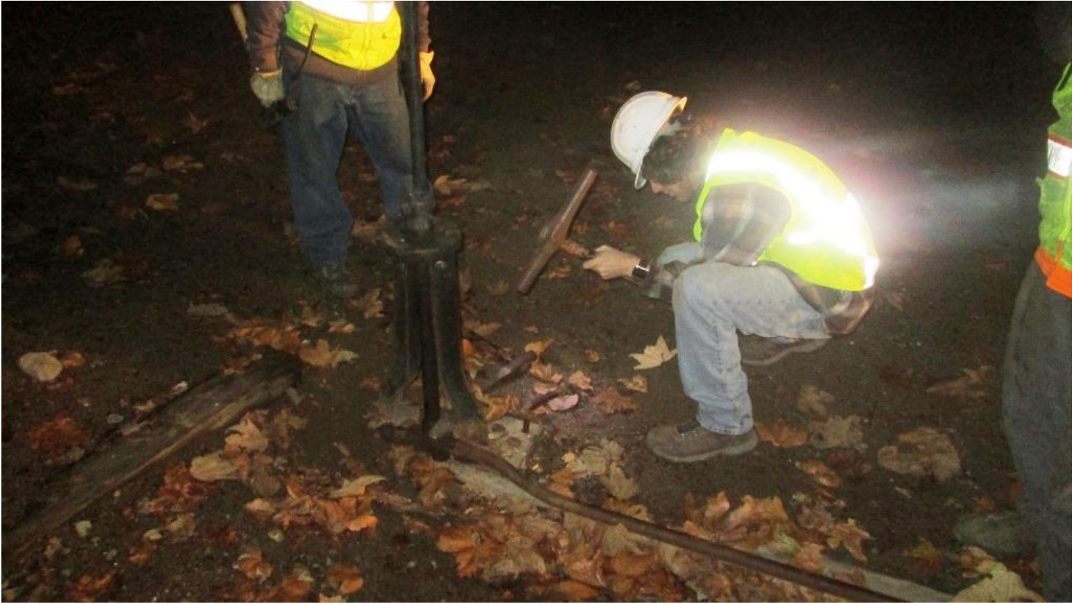
Matt drives spikes into the newly plugged spike-holes at the switch
