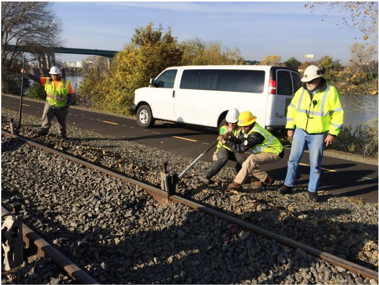
Sometimes, it takes a little effort to raise the track as Matt and Chris M. demonstrate...
