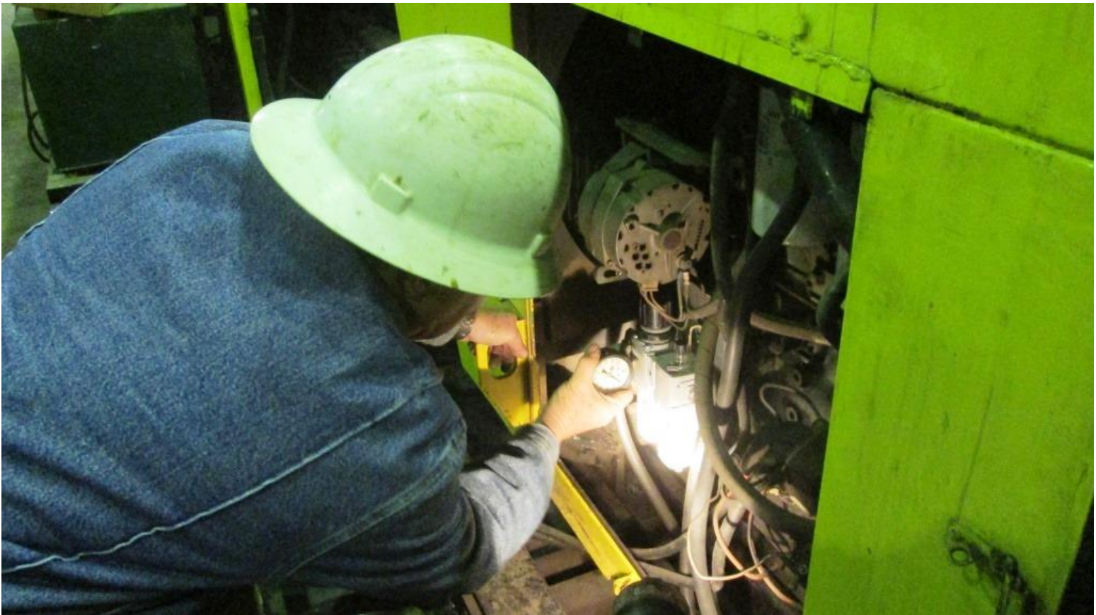
Mike H. checks air-pressure at various valves as he trouble-shoots the tie-shear's problem
