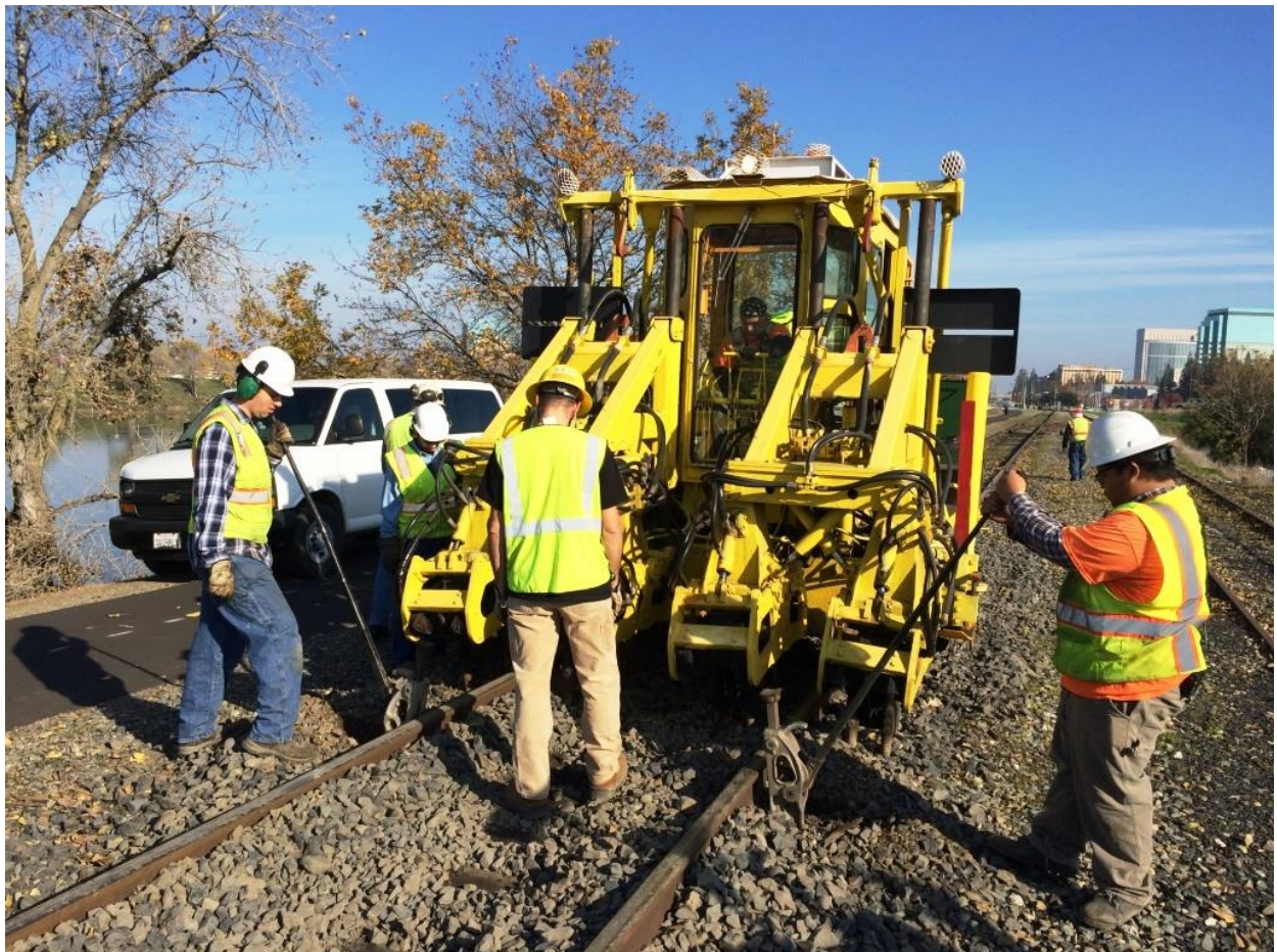
Chris M. takes over guiding the tamper as Weston and Anthony prepare to pull jacks
