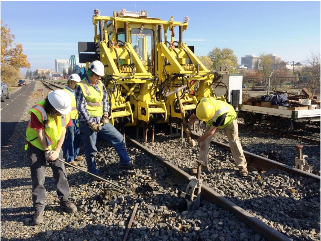
Track triage: Matt nips up a tie (that didn't lift when the rail was raised) as Chris M. re-spikes it
