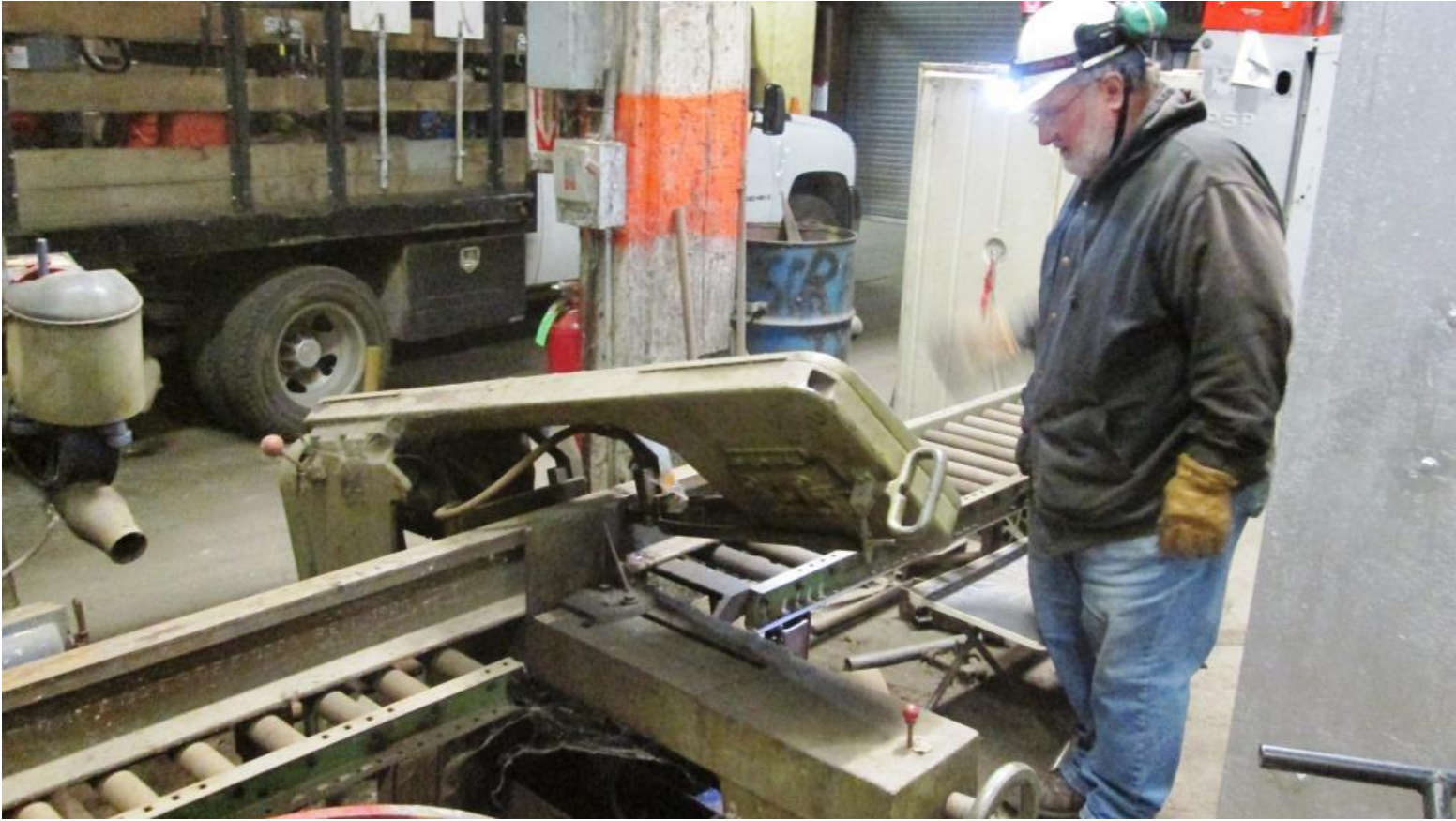
Frank uses the rail-saw to cut the rail being milled for replacing the cracked wing-rail to its proper length
