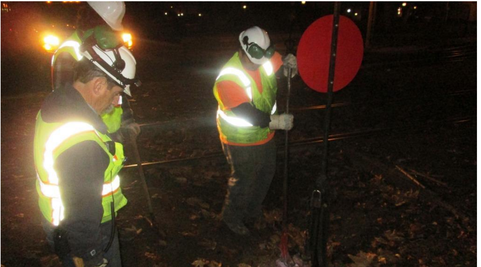
Anthony pulls spikes at Switch 2 as Joe and Matt stand ready to plug and re-spike the stand
