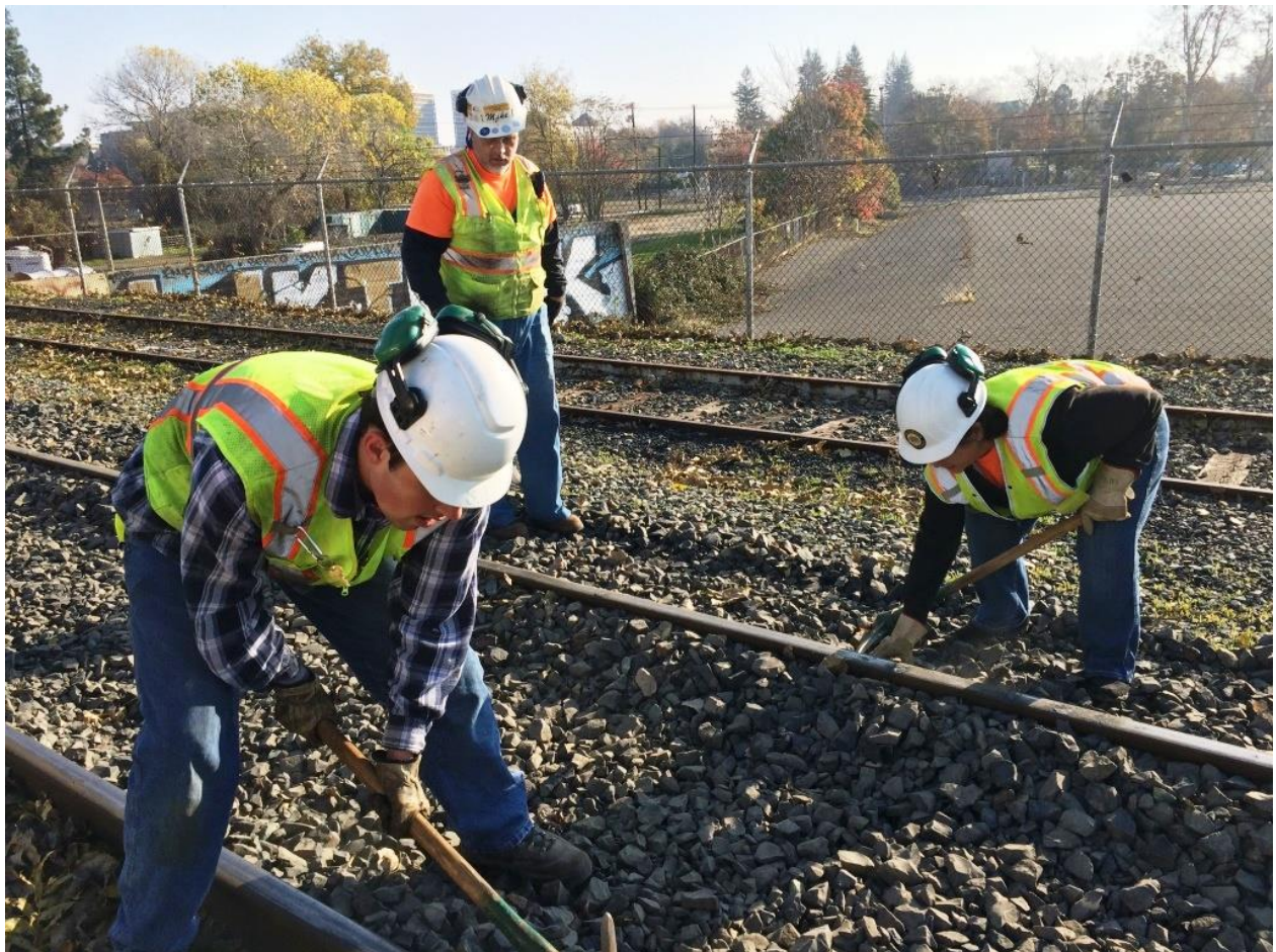
Weston and Pam dig pockets under the rails for jacks to be inserted
